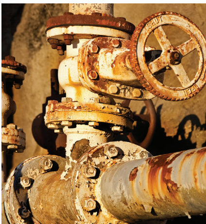
Flange Corrosion
